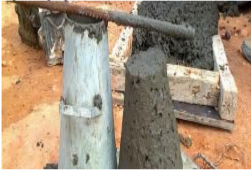
Figure3.a Slump test preparation
